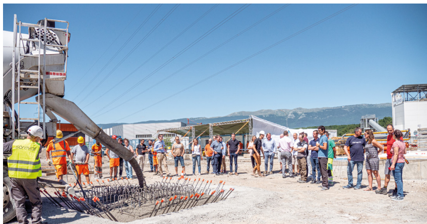
Concrete covering the capsule
